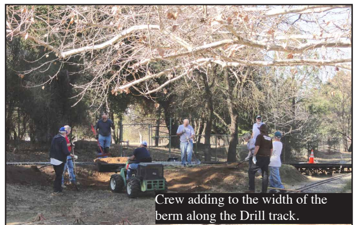
Dick Patton and Jack Slavin installing new end of track bumper.
