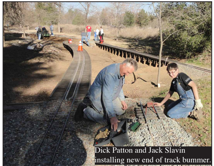
Drill track is being re-ballast after re-alignment away from main line.
