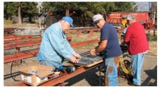
Tie plate gang. Tie plates were preset to gauge on plastic ties.
